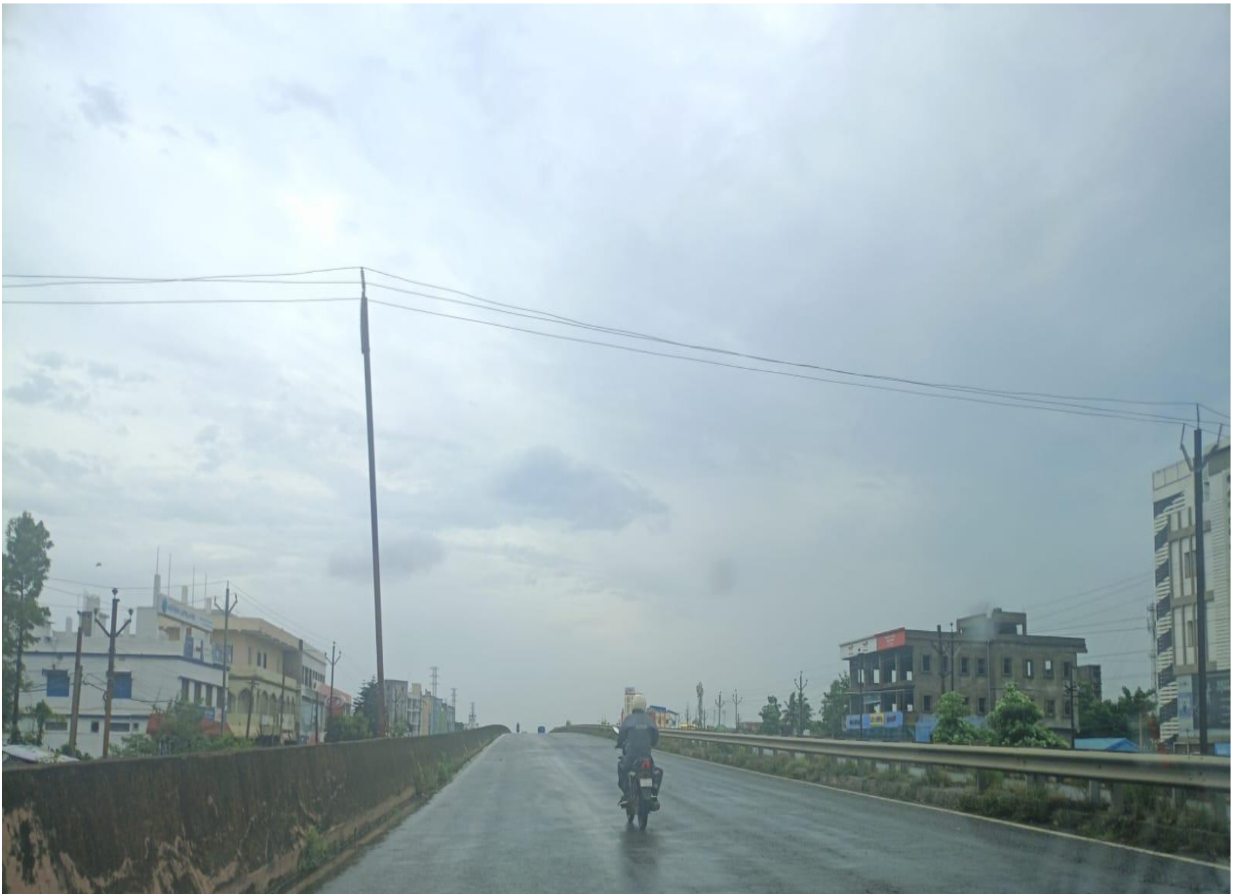
IMAGE: Bridge; Risk Level: High; Coordinates: 21.511436 , 86.892188
