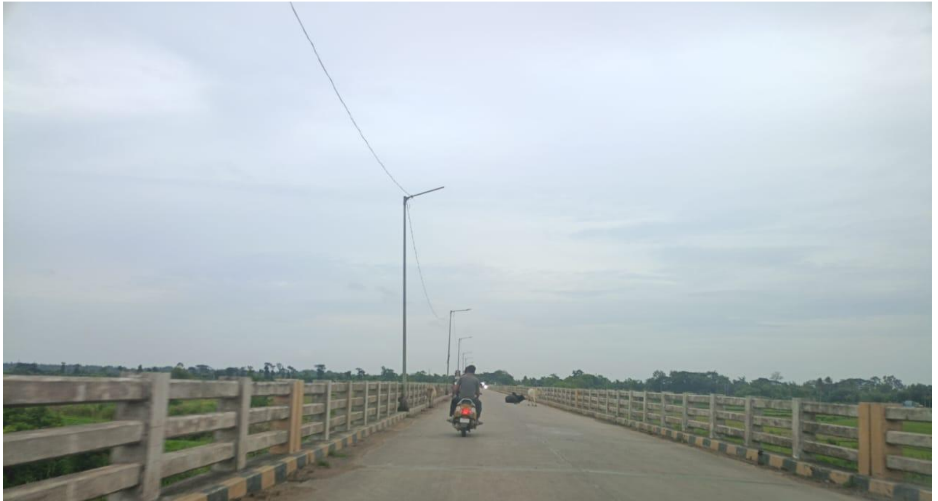
IMAGE: BRIDGE ; Risk Level: High ; Coordinates: 21.700371, 87.409532
